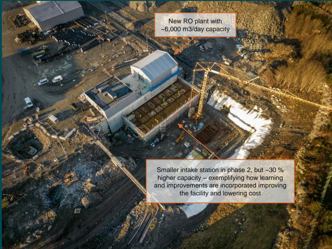
Concrete works for intake station (January 2025)
