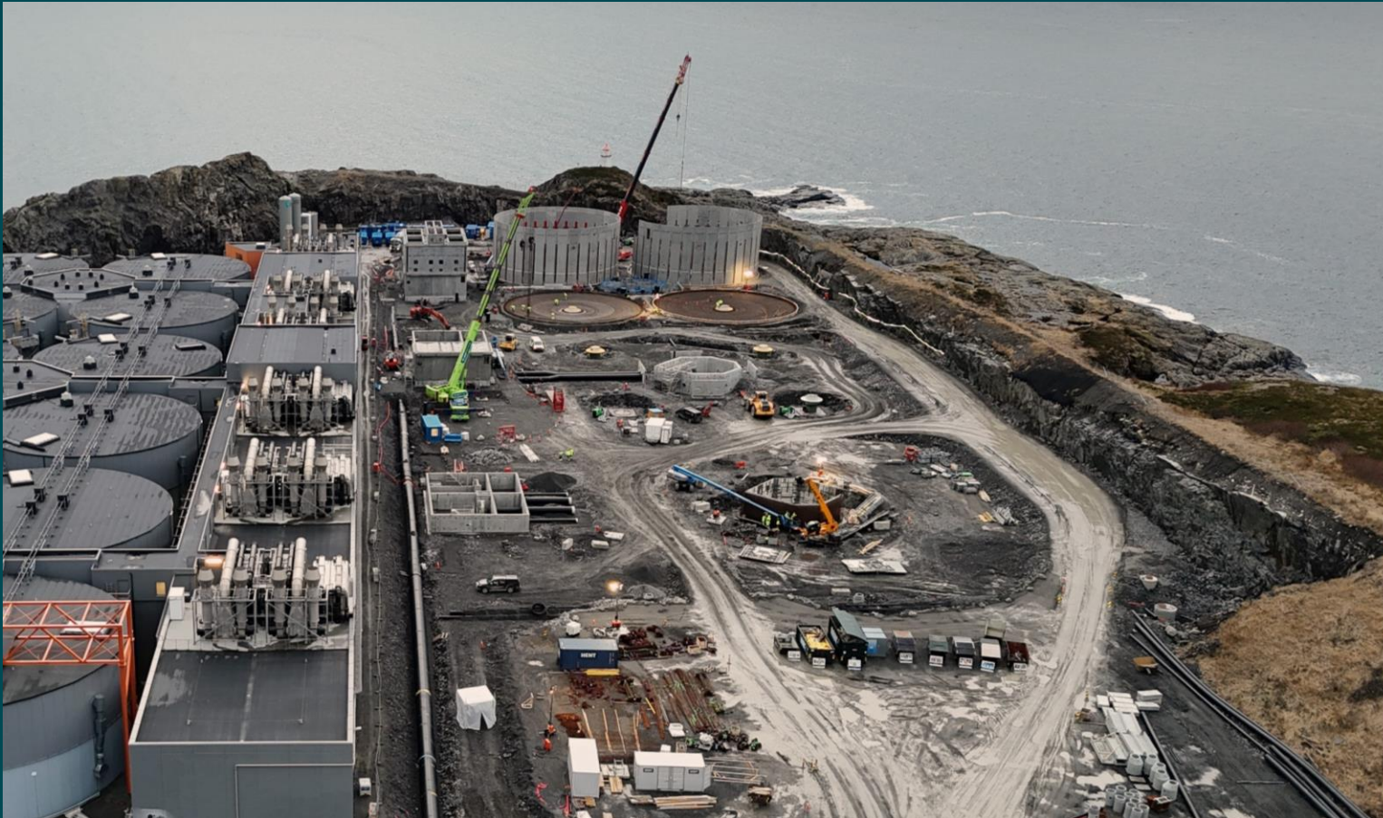
Tank installations well underway (February 2025)
