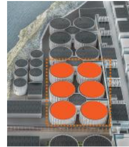
RAS Recirculating aquaculture system
